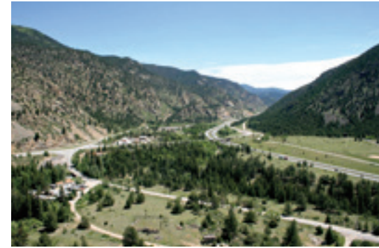
TRANSIT PLAN As part of its work with parent firm Typsa, AZTEC is creating a feasibility study for Colorado DOT’s proposed high-speed rail from Denver to surrounding areas.
